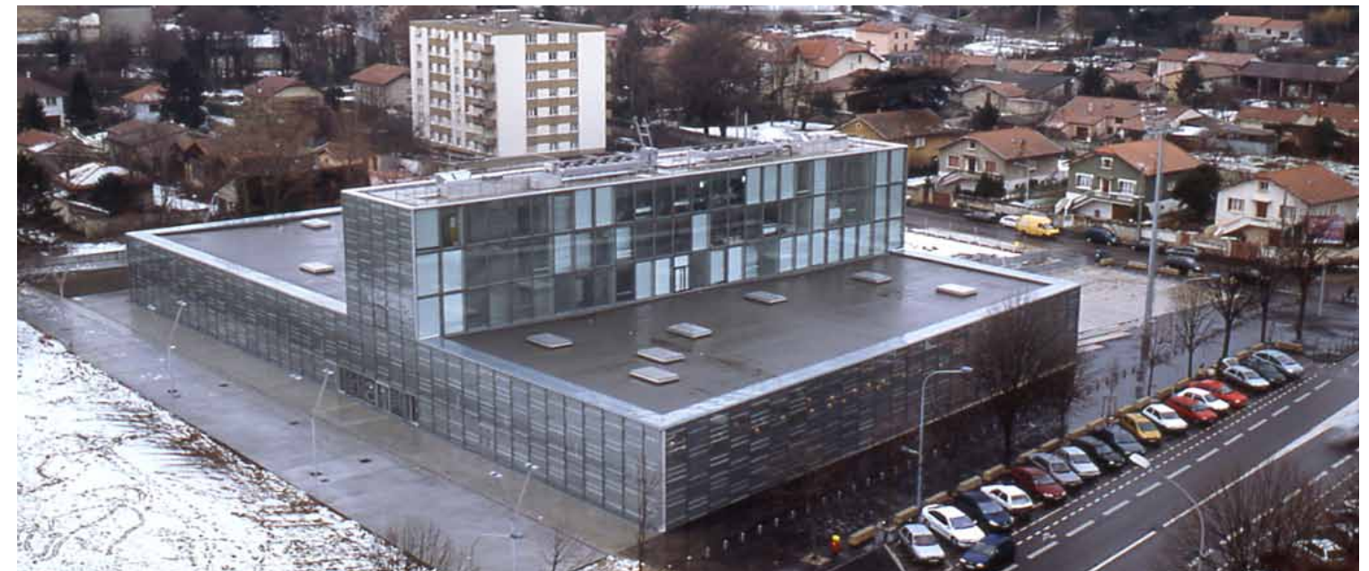
aerial view, Media Library, Vénissieux, France
