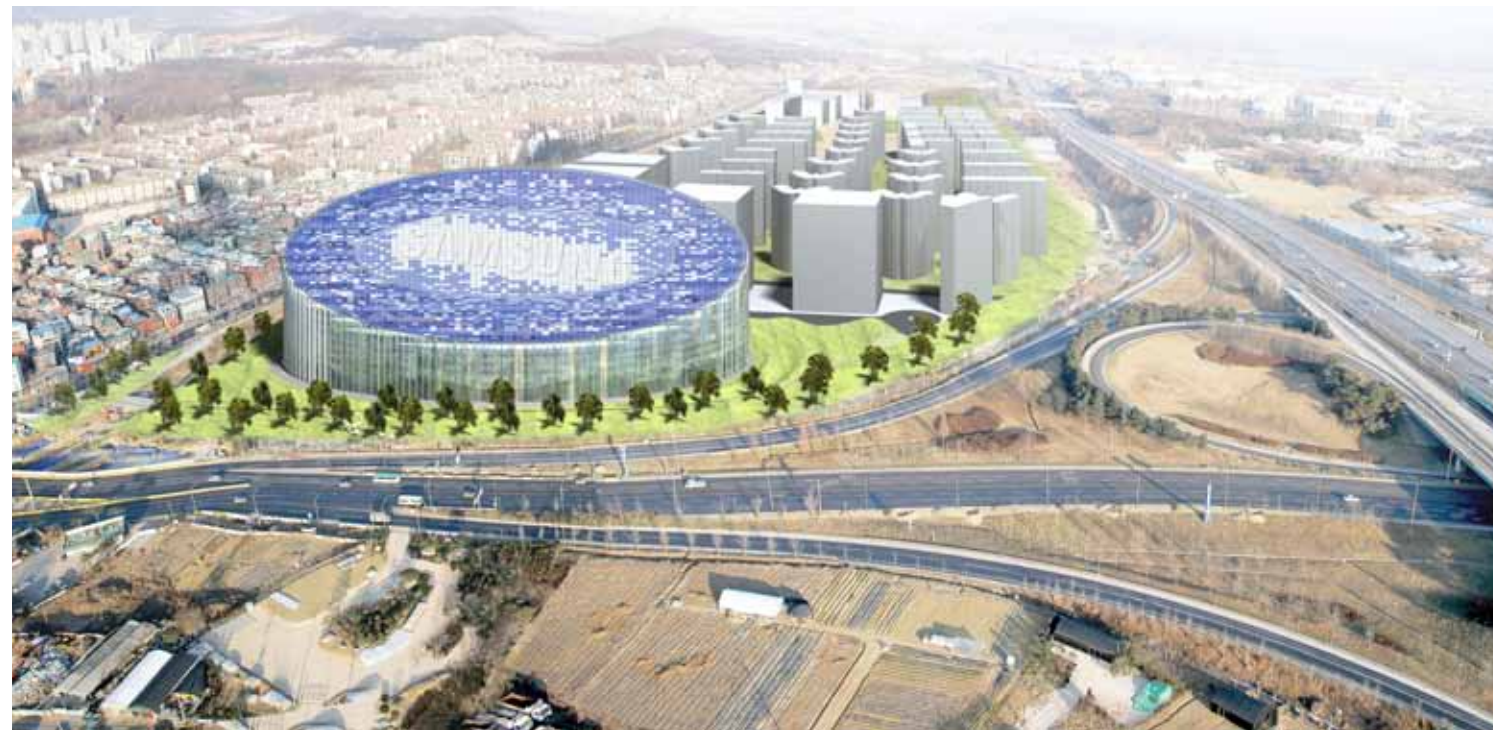
aerial view, Samsung Engineering Center, Seoul, Korea
