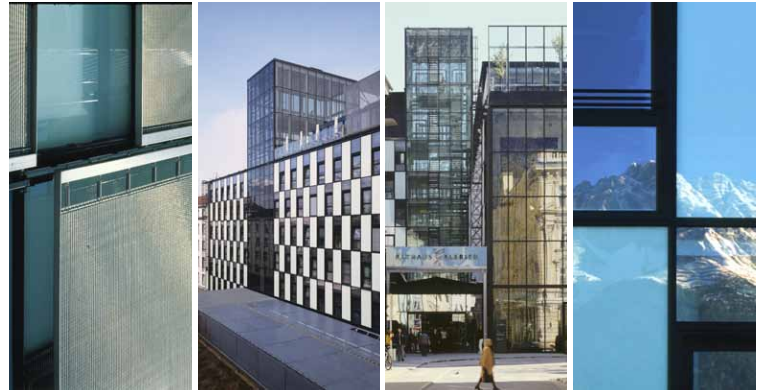
facade details, Town Hall district, Innsbruck, Austria
